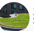
The green roof over the chapel retains water and reduces heat to increase energy efficiency.
